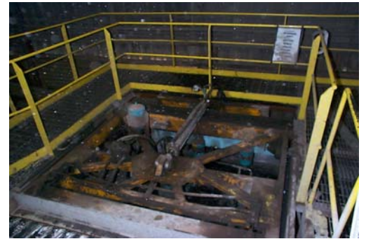
OLD BRICK SLUG PUSHER
